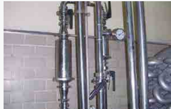
Milk Production Line Line Strainer (Material : SUS316L) Hole Diameter : 70µm, Plate Thickness : 0.5mm (0.019 inch)
